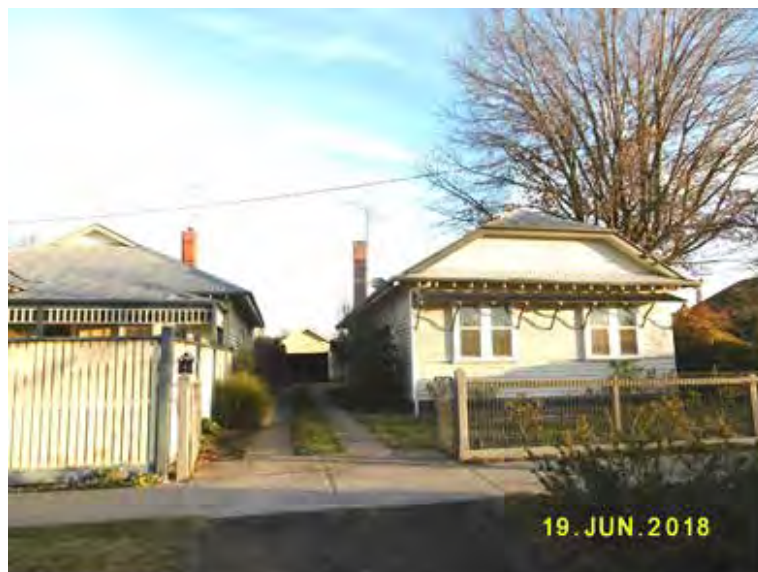
Figure 1: Existing site context (Site inspection photo)
