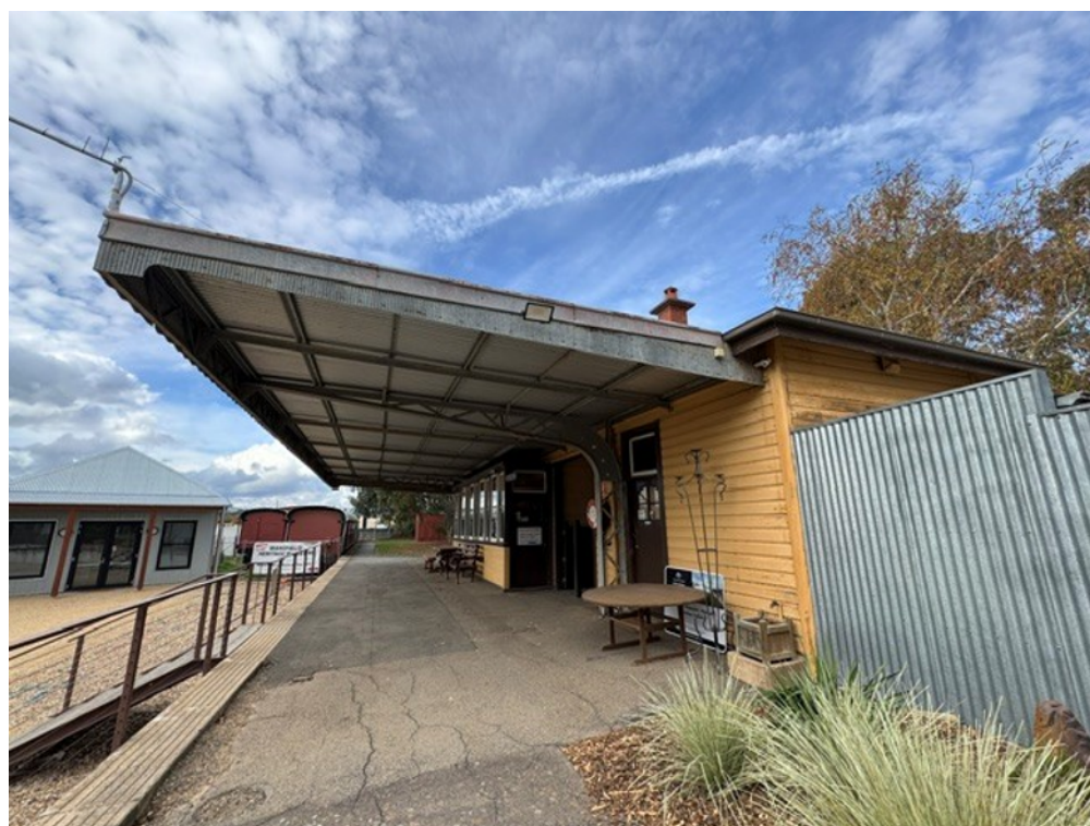
Figure 3 – Back and Platform of Station Building
