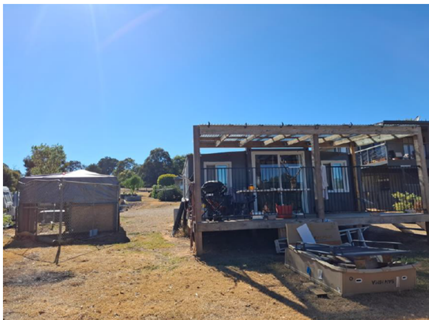
Figure 6: View looking towards the west elevation / front entrance of the habitable outbuilding, February 2025
