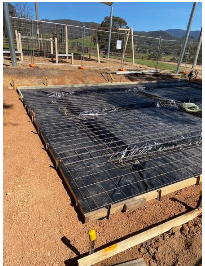
Picture: Site cut and slab preparation for Macs Cove BBQ shelter
