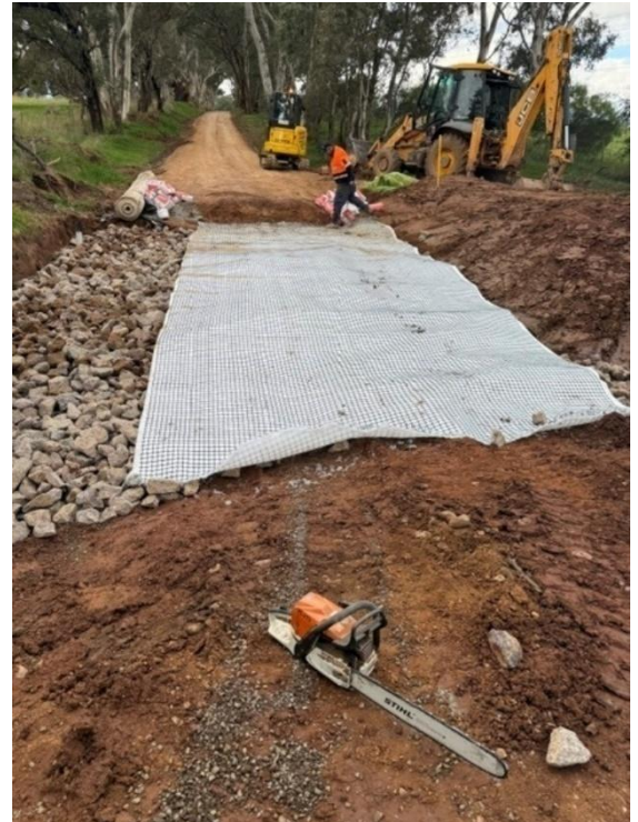
Image: Works to rectify spring under Tabletop Road
