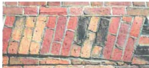
Examples of lintel detailing
