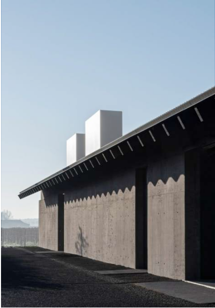
EXAGGERATED METAL ROOF OVERHANG
