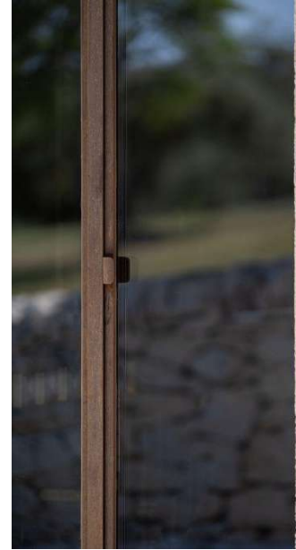
WEATHERED STEEL FRAMES TO EXTERNAL GLAZING
