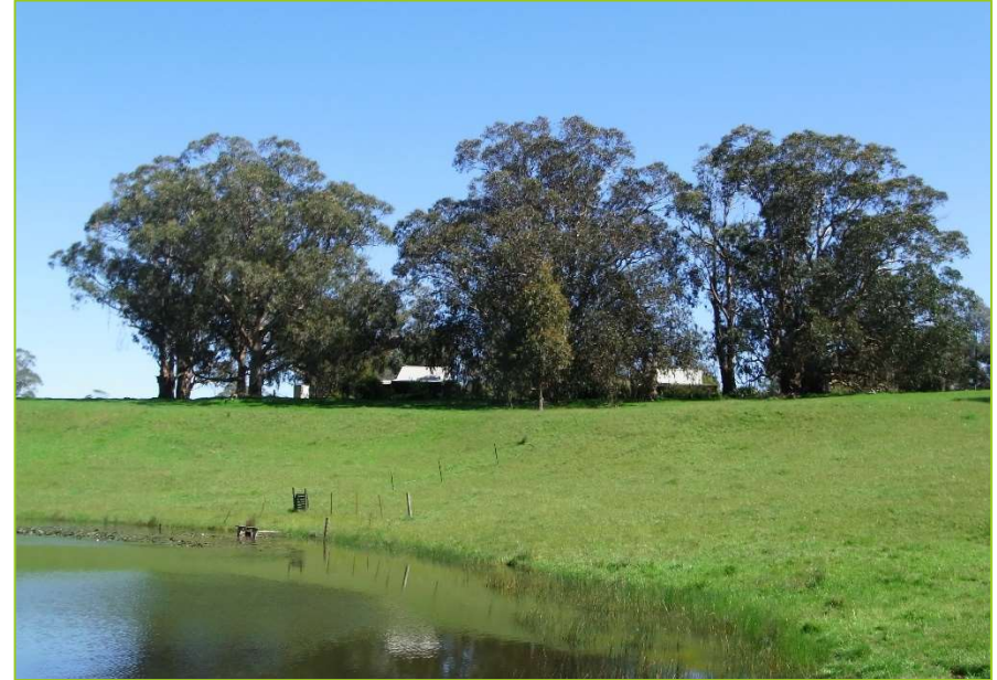
6. Edge of dam, with large old trees and cottages behind, from SE.
