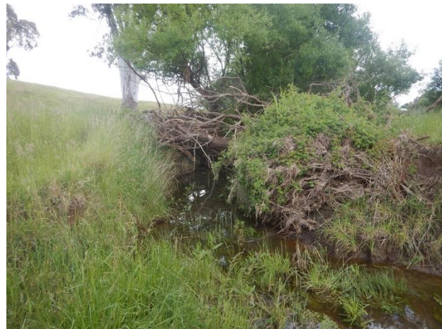
Photograph 6 Owens Creek showing erosion of banks (D.Carpenter, 16/11/2021, facing south)
