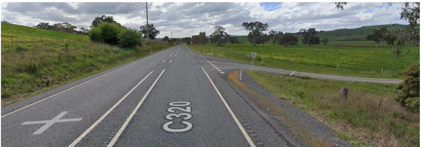
Figure 5: Ingomar Road intersection, source: Google Street View
