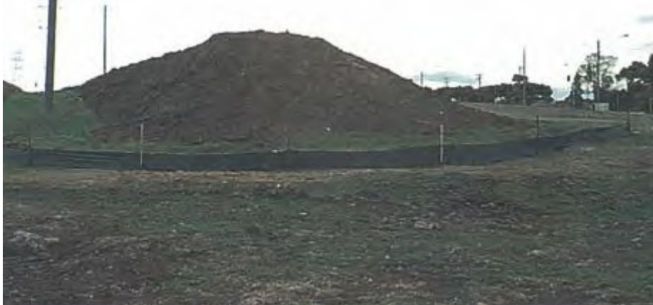
Topsoil stock pile surrounded by a silt fence
