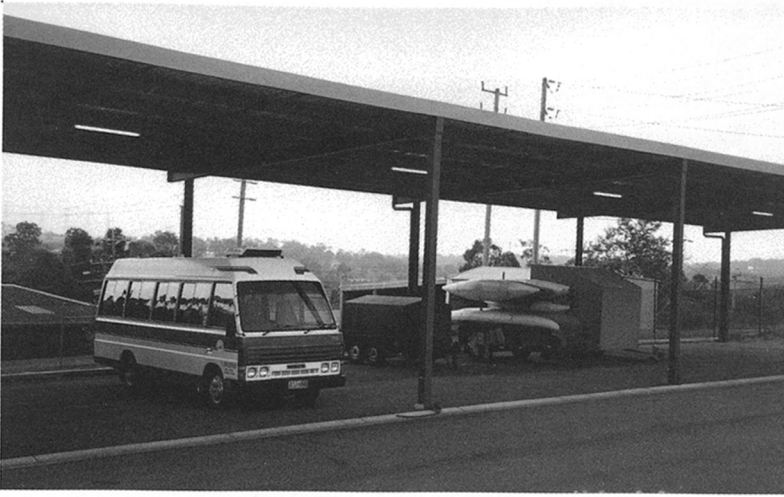
Figure 6.2 A temporary storage facility, undercover and with a spoon drain to redirect surface flow (City of Manningham).
