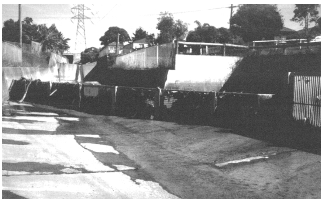
Figure 7.12 Trash rack (Cup and Saucer Creek, Sydney).
