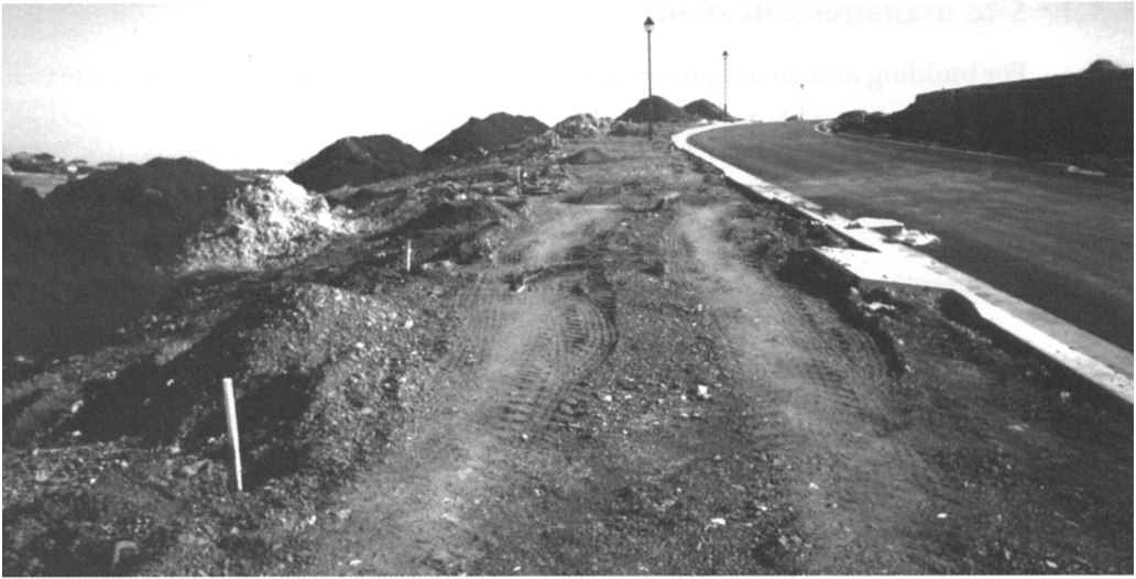
Figure 6.7 Land development results in significant vegetation removal and soil disturbance.
