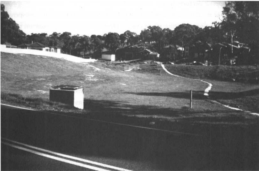
Figure 7.29 Extended detention basin.
