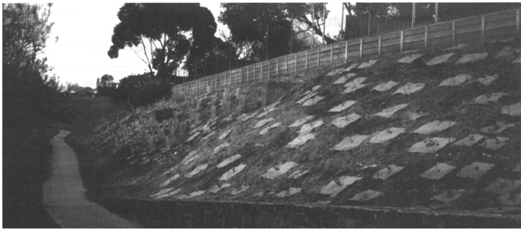
Figure 6.10 Stabilisation and revegetation protect soils from erosion.
