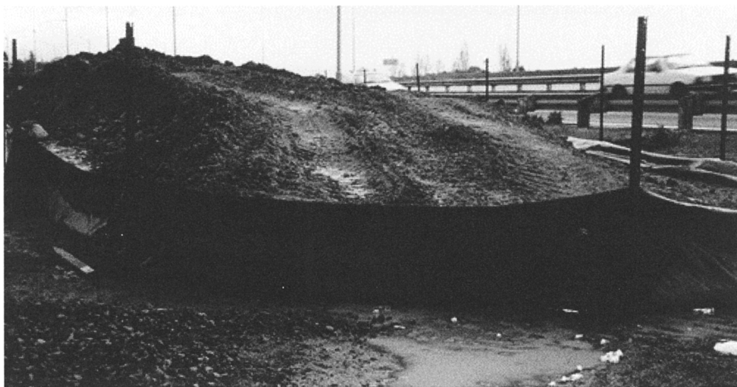
Figure 6.13 A silt fence around a stockpile.
