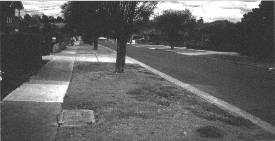
Prospect Street looking west along drainage path.
