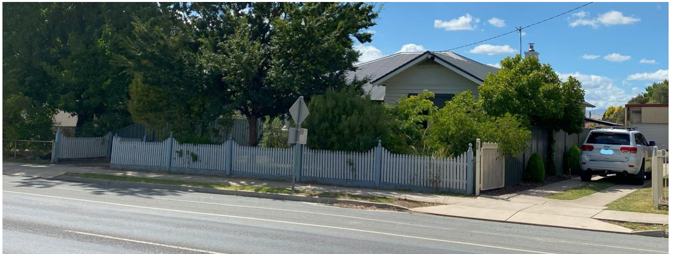
Adjacent property – 30 Chenery Street (northern boundary)
