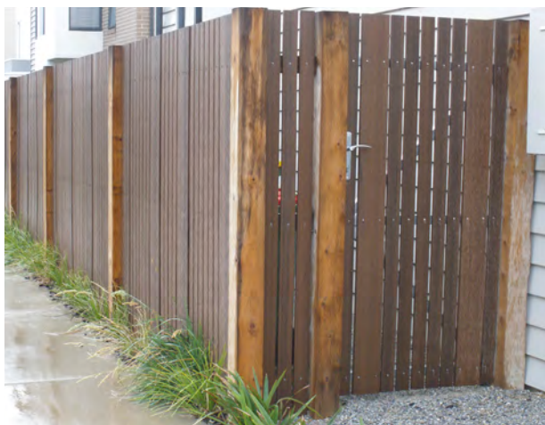
Figure 25 Example of waste storage area screening.
