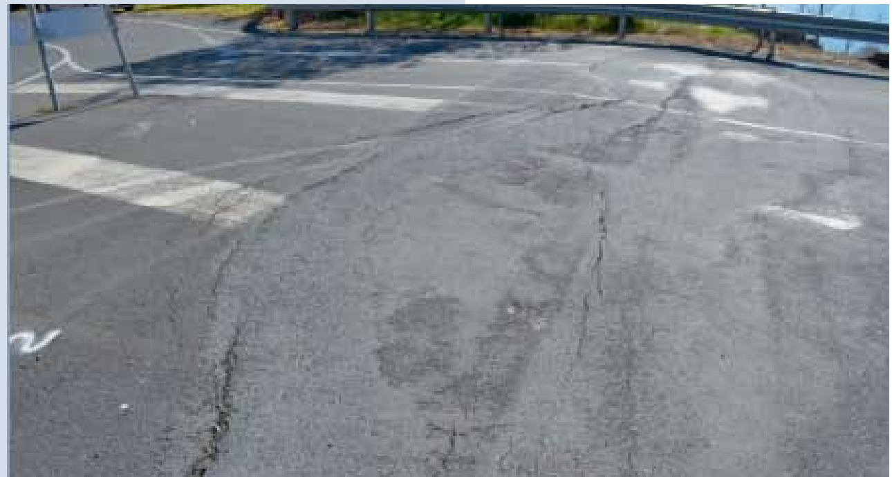
The existing car park adjacent to the ramp is showing signs of pavement distress.
