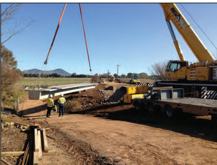
Top: Eildon-Jamieson Road safety installation; Mansfield Memorial Gates Above: A Dead Horse Lane Bridge Heavy Vehicle Bypass.
