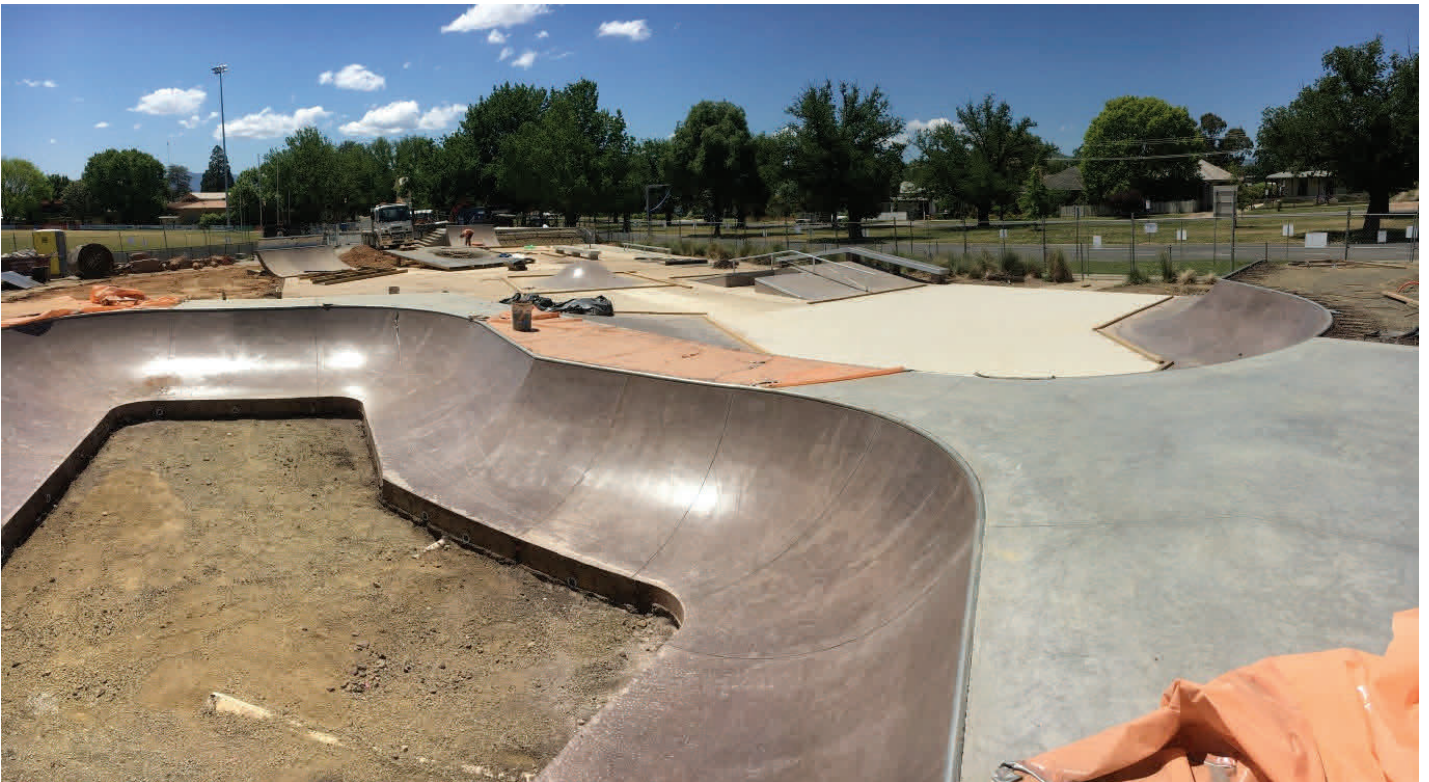
Top: Erril Street Rejuvenation and Activation project Above: Mansfield Skate Park under construction.
