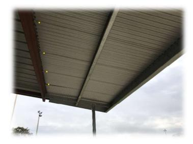
The underside of the main awning is open and unlined which provides perching points for birds. There is a health risk associated with the extent of bird droppings present. Bird droppings not captured in this photograph.
